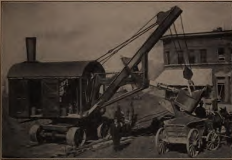
Thew Revolving Steam Shovel. Figure 27.
